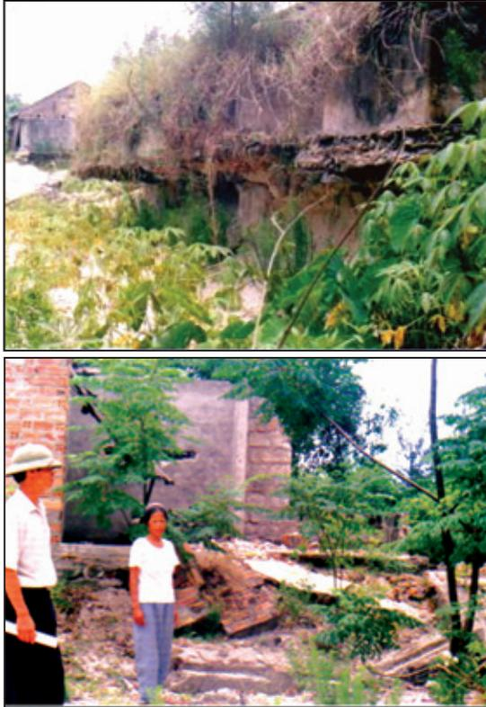
**Photo 2: Sand flow in Le Thuy (Quang Binh) in 1999: the foundation of a pumping station (upper); this woman's three-room brick house is collapsing because sand has been blown from foundation (lower).**
